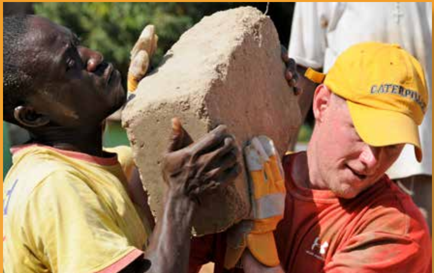
Building a new library in Ghana.
