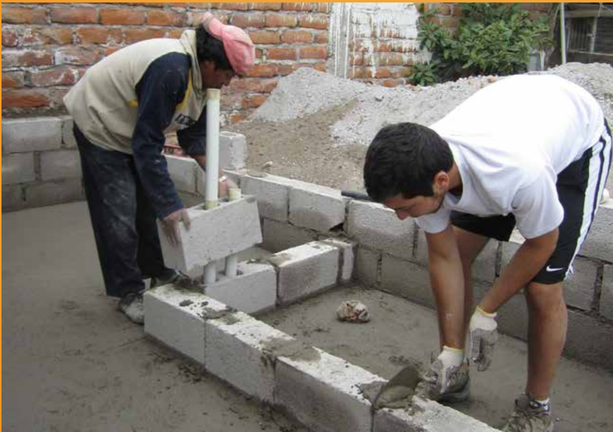
Volunteer helping construct bathroom facility at a child care facility in Ecuador.
